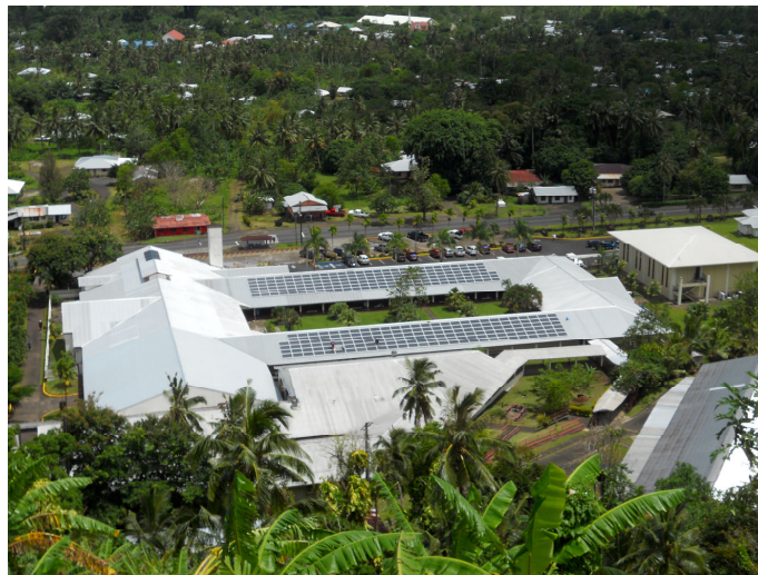
New solar panels on ASCC rooftops
